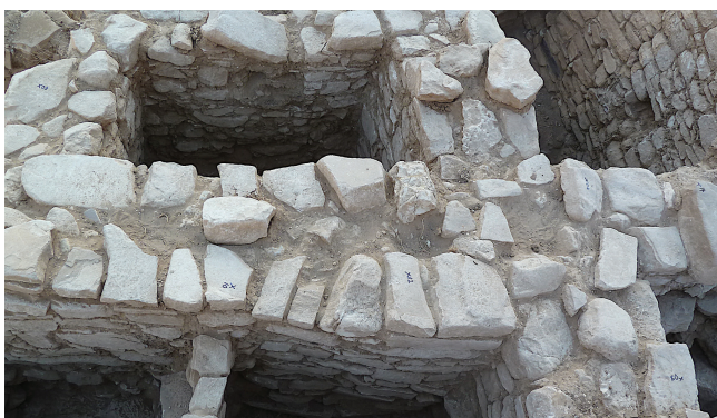
Fig. 7 BNR42-44, Wall Loc. B11:2b: Example of an eroded horizontal section through a standard double-faced wall in Ba`ja. (Photo: H.G.K. Gebel)
