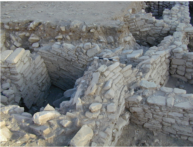
Fig. 5 Area B-South, Squares B84-85: Leaning, tumbling and twisted walls resulting most likely from a quake impact. View from south in 2003. (Photo: H.G.K. Gebel)
