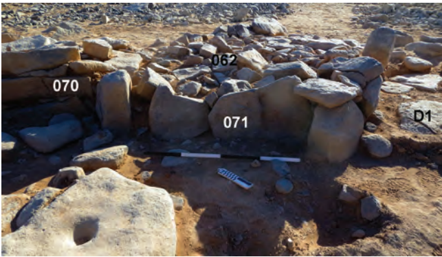
Fig. 12 Renovations in the north wall of W-80. An opening was made in wall 070, then blocked sometime later using basalt slabs placed on edge (071), creating doorway 069 at the same time. Platform 062 was built to the north of 070. The original eastern wall 019 of W-80 is just off the photo to the right. (Photo: G. Rollefson)
