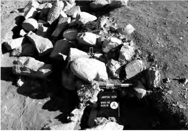
Fig. 12 Wadi Ruweishid ash-Sharqi Barrage 2: A close-up view of the protruded reinforcement wall at the converging point (from S).
