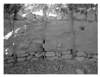
Fig. 1 Interior view of one of the experimental reconstructions illustrating the extent of damage from flooding.
