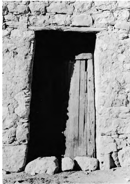
Plate 69.B. Door with wooden lintel. Example from Old Basta. 1987
