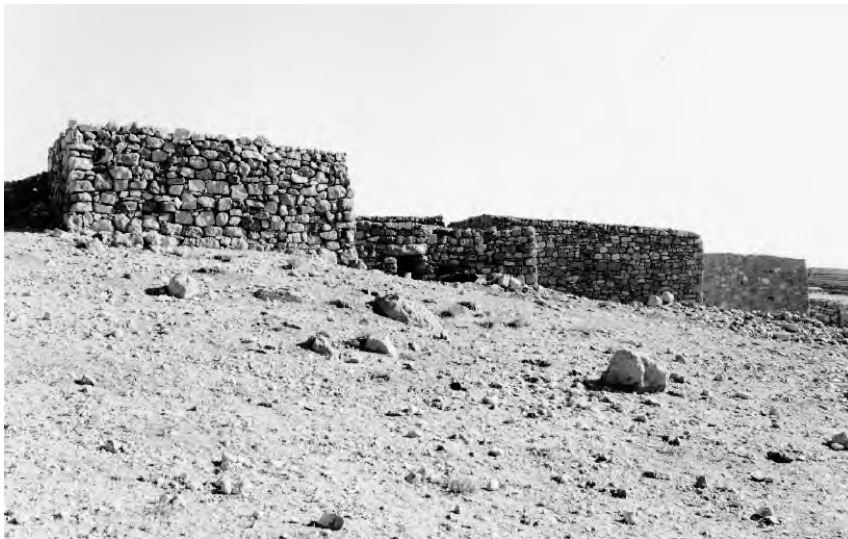
Plate 71.C. Old Basta. Windowless exterior walls. 1987.
