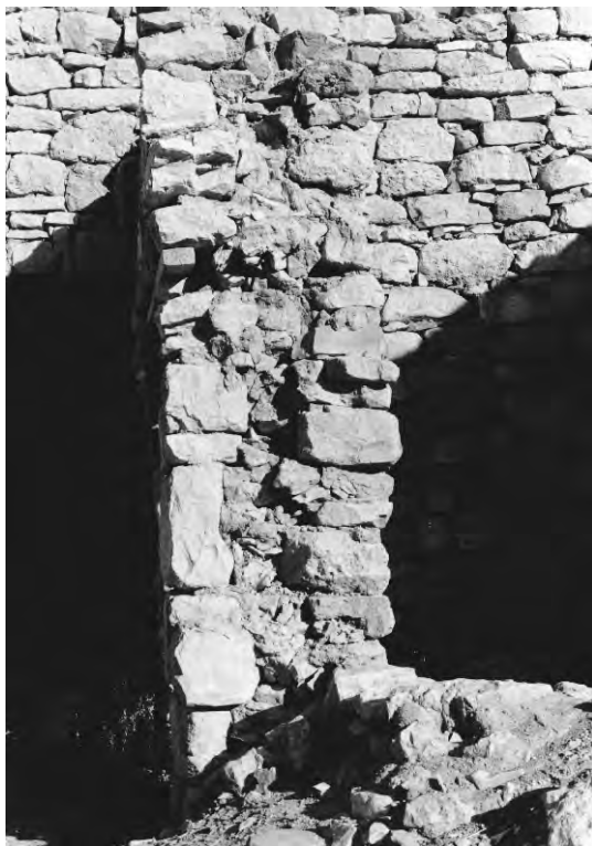
Plate 69.C. Double- faced wall with rubble fill. Example from Old Basta. 1987.
