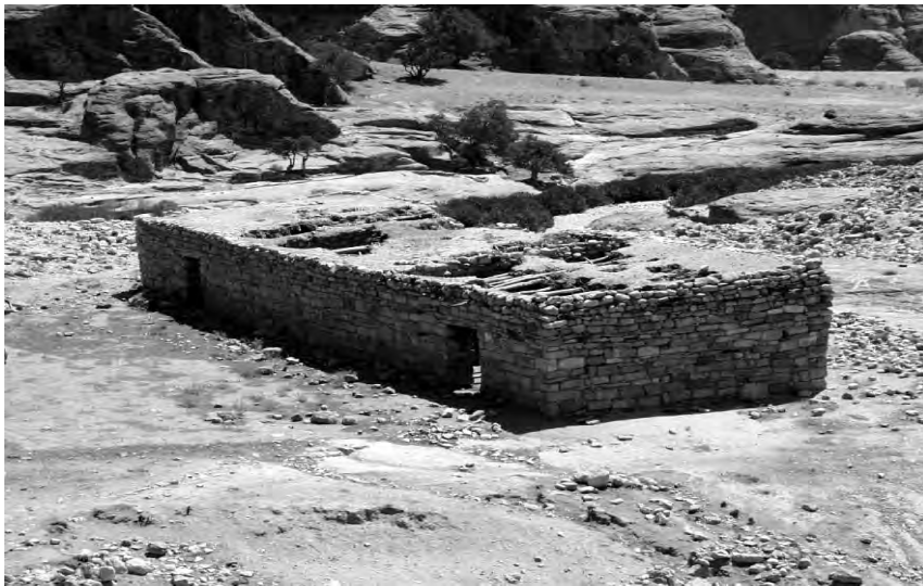
Plate 72.B. Exterior wall with partly preserved mud plaster. Example from Old Basta. 1987.
