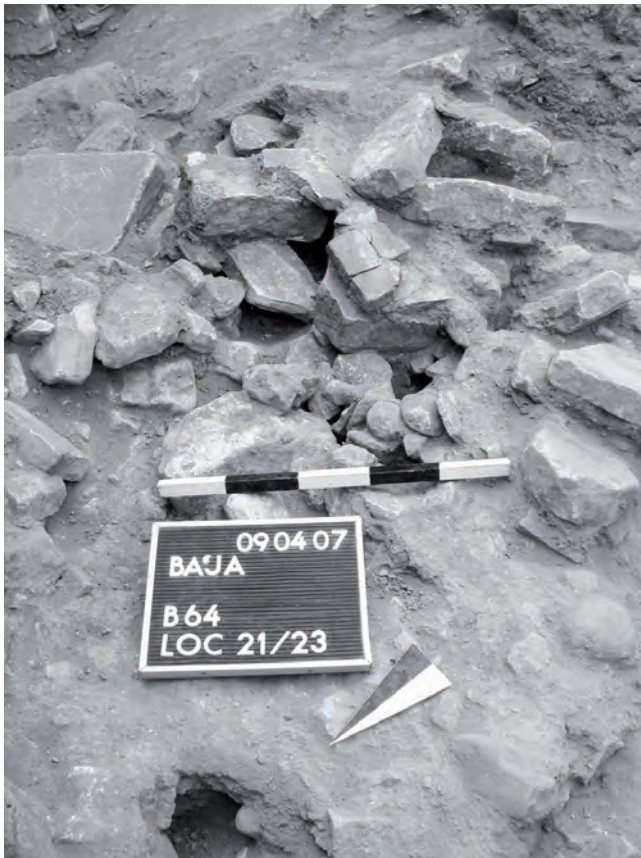
Fig. 21 Ba'ja, Area B-South, Square B64-South, Loci 21 and 23: LPPNB wall rubble found with air pockets (earthquake damage?)
