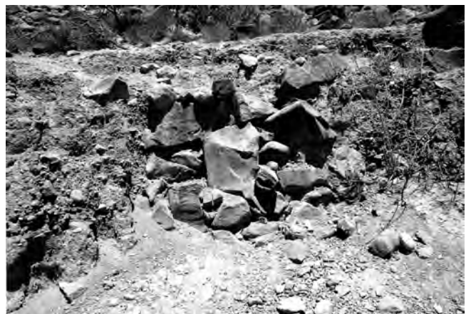
Fig. 5 A close-up view of the barrage wall at the northern bank (looking N).
